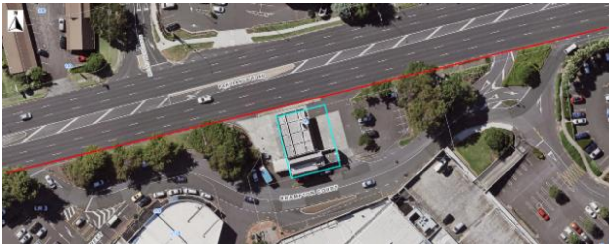
Figure 82: Pakuranga Rd longitudinal drainage works and GAS service station (blue outline)
