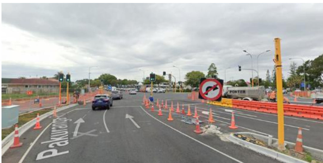
Figure 20: Pakuranga Rd / Ti Rakau Dr intersection, looking eastbound on Pakuranga Rd (source: Google Street View, Feb 2021)
